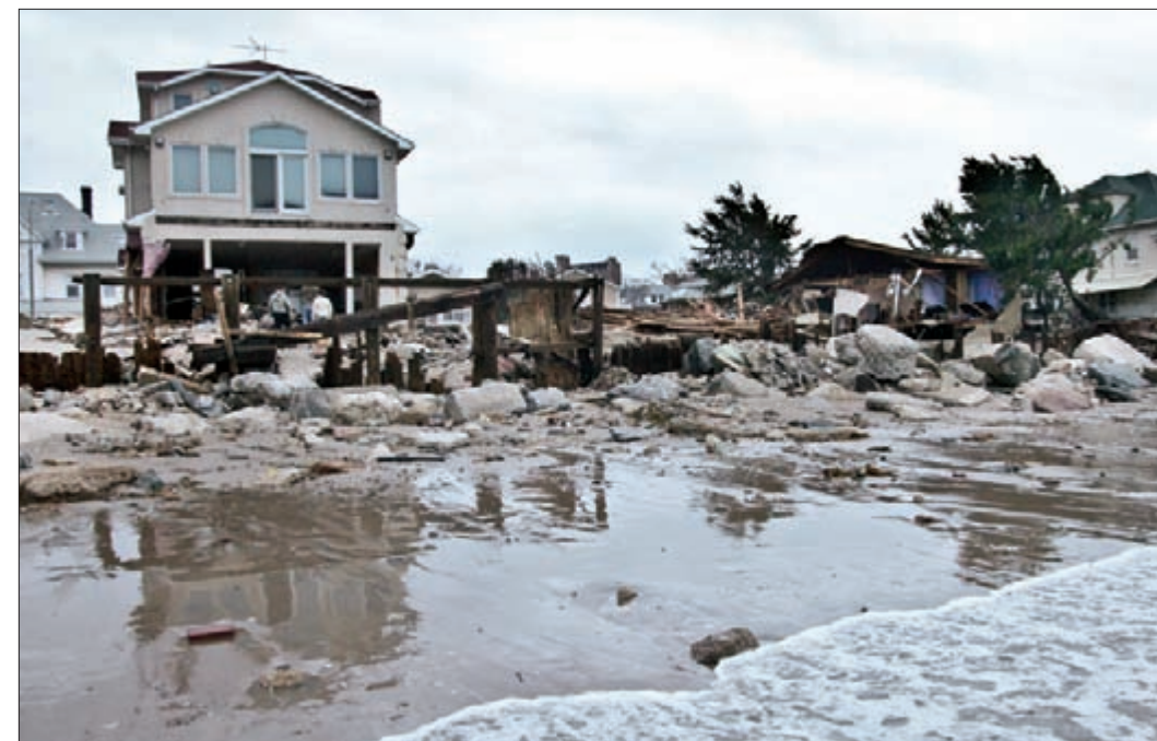
New York's coastal areas, including Coney Island and the Rockaway Peninsula, suffered tremendous damage from Hurricane Sandy. In Coney Island's Sea Gate community, many beachfront homes were battered by the storm surge.
